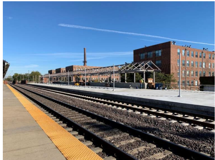
Track level construction of platform and canopy at Ravenswood Station.
