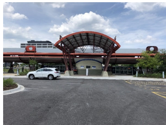
On-site photo of the Pace Northwest Transfer Center.
