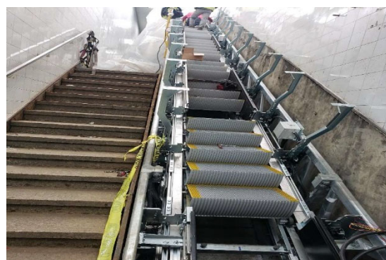
New escalator installation.
