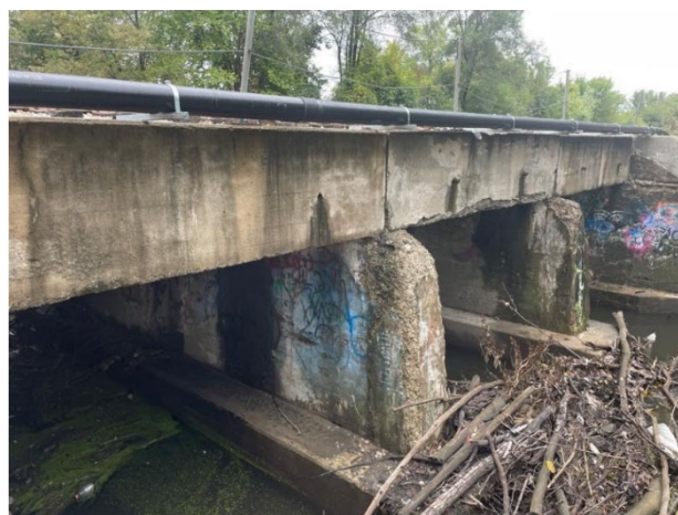
Current condition of the Stoney Creek Bridge
