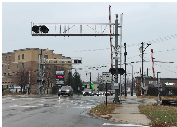
Picture of existing Metra grade crossing.
