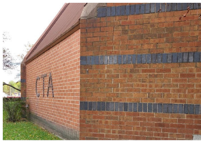
Kedzie Bus Garage façade existing condition.
