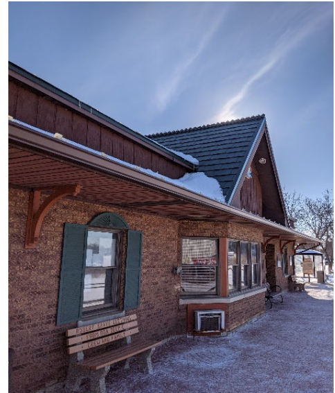
Existing Fox Lake crew facility
