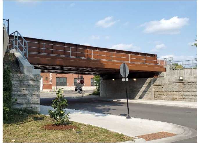
Completed bridge over Berteau Ave. along UP-North line.
