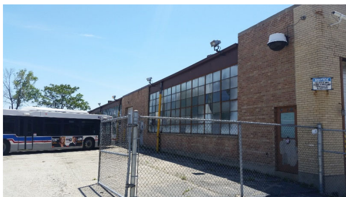
Existing Forest Glen Building.
