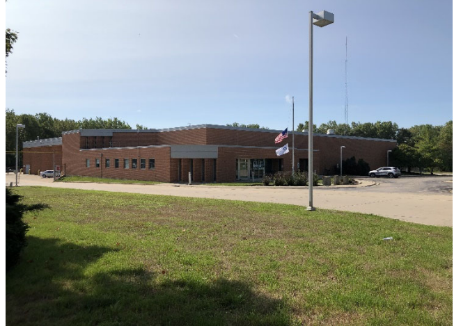
Existing River Division bus garage.
